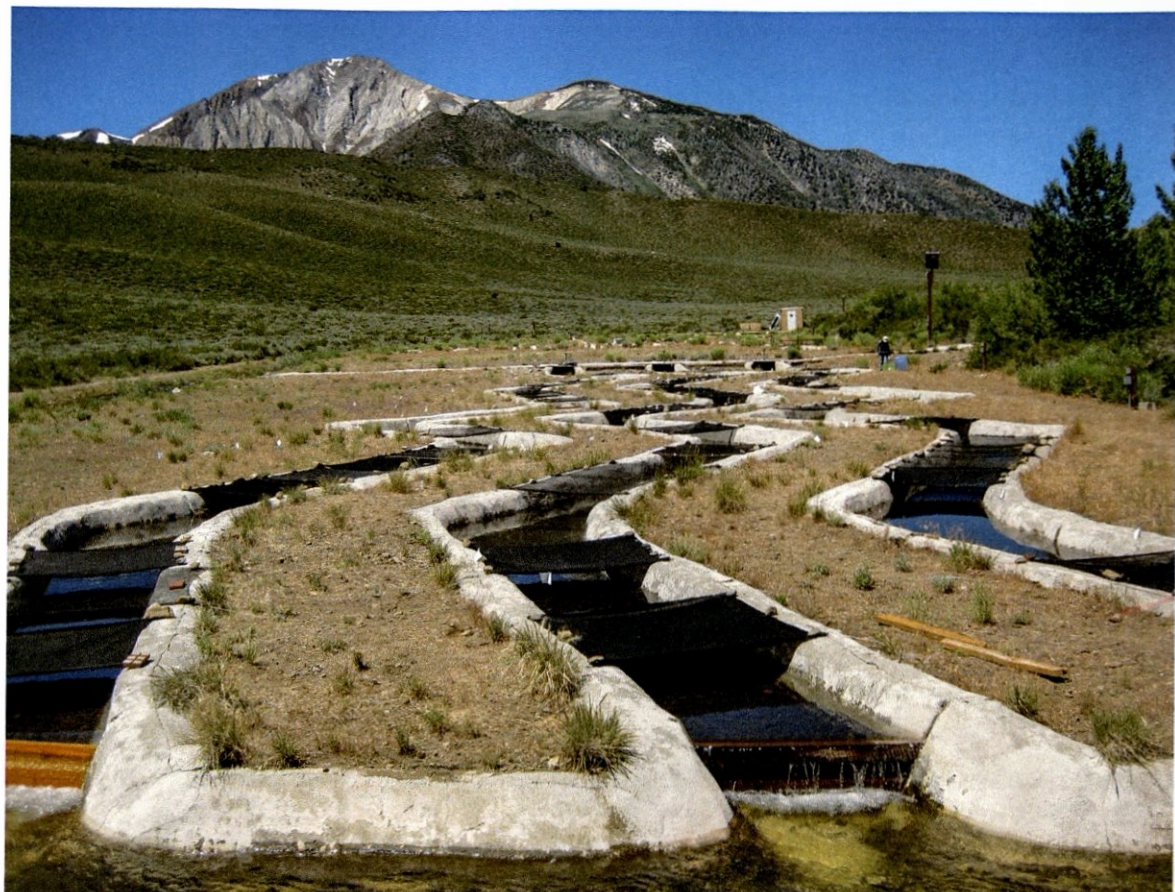
FIGURE 8.8 The Sierra Nevada Aquatic Research Laboratory contains outstanding research facilities, including a unique network of experimental streams. Photograph by Emily Peffer Zefferman.
